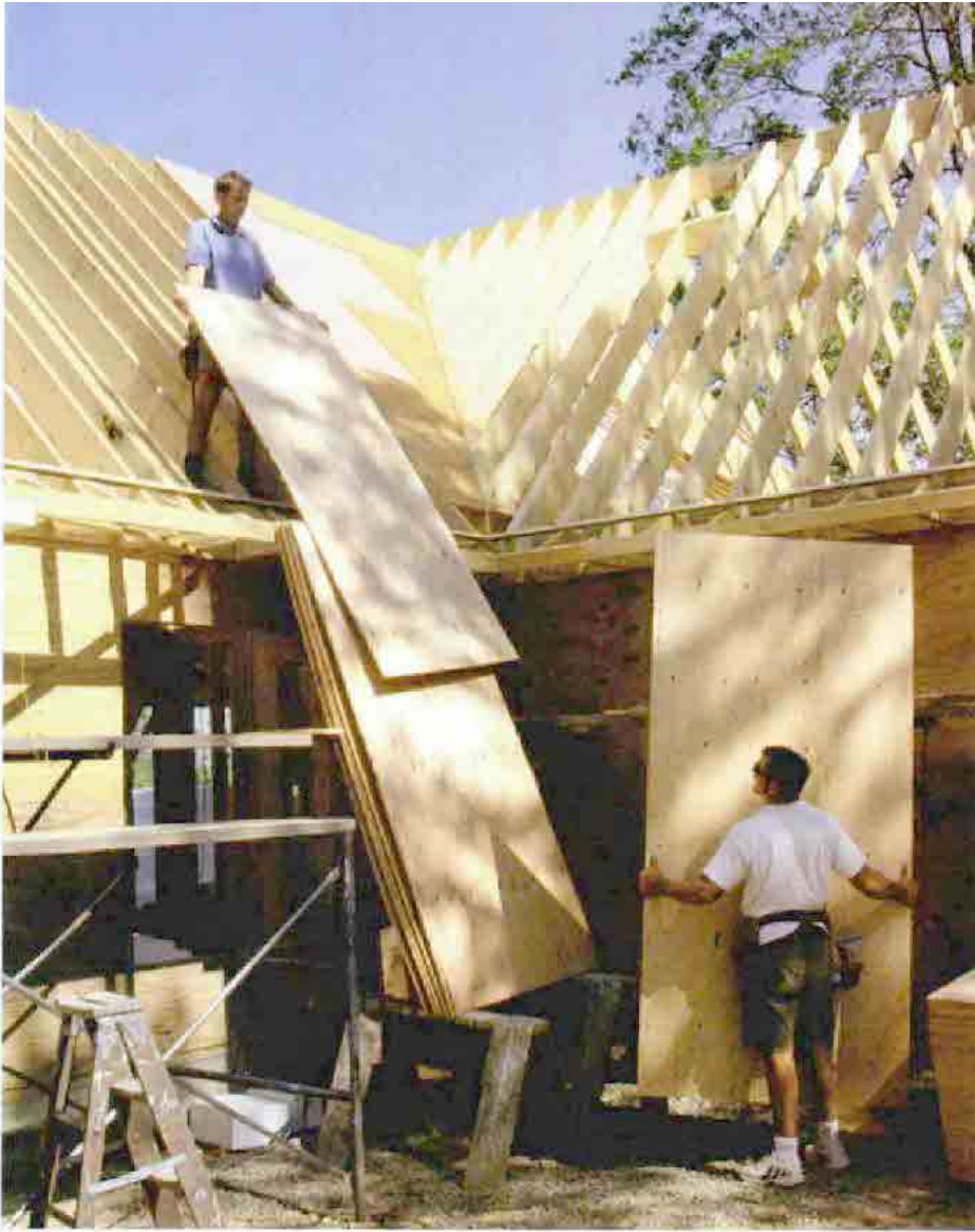
Sawhorses make for easy picking. The easiest way to get the sheathing onto the roof of a single-story house is to lean the sheets against the fascia on top of two sawhorses.
